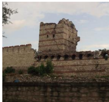
Figure 2 – One of the Towers of Land Walls with a massive crack on it Latitude 41 00 45.92 N Longitude 28 55 19.77 E (WGS-84)
