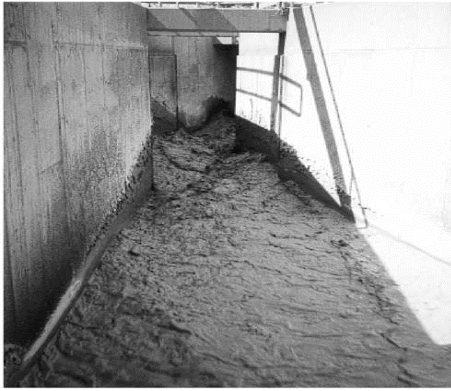
FIGURE 2 Large concrete structures offer a method of conveying large quantities of slurry. This structure was built to convey 150,000 tons per day of soft high clay tailings at a Peruvian copper mine. (BAHA E. ABULNAGA, PE.,2002, p. 6.2)
